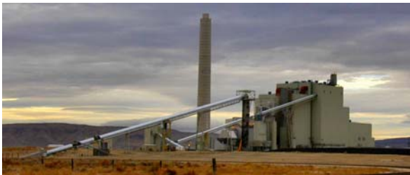
Newmont TS Power Plant
